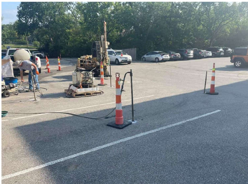
Figure 4. One of the ISCO injections
